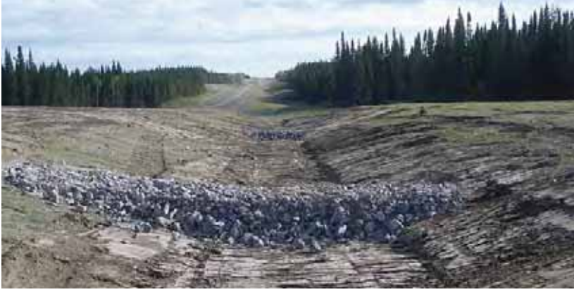
Rock check dam installed in ditch along access road.
